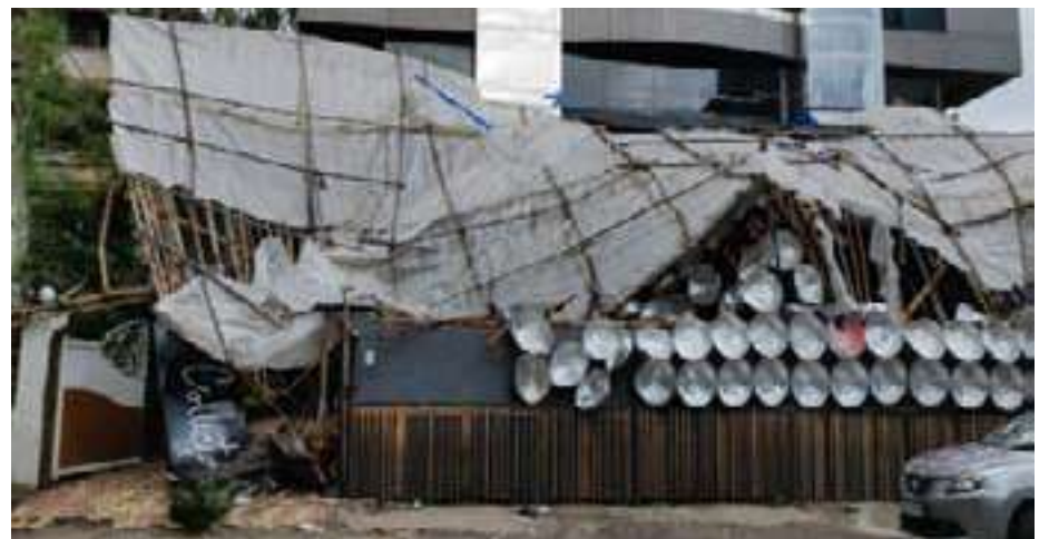
Various encroachments were demolished by the PMC in Viman Nagar
