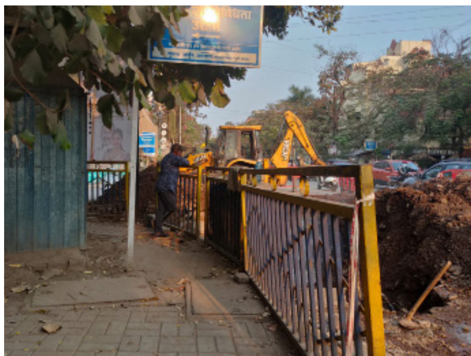
A pavement next to a road under construction in Viman Nagar
